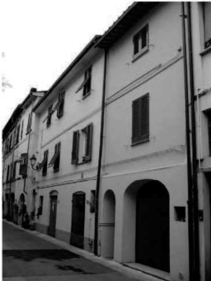
D 5 via Cavour
