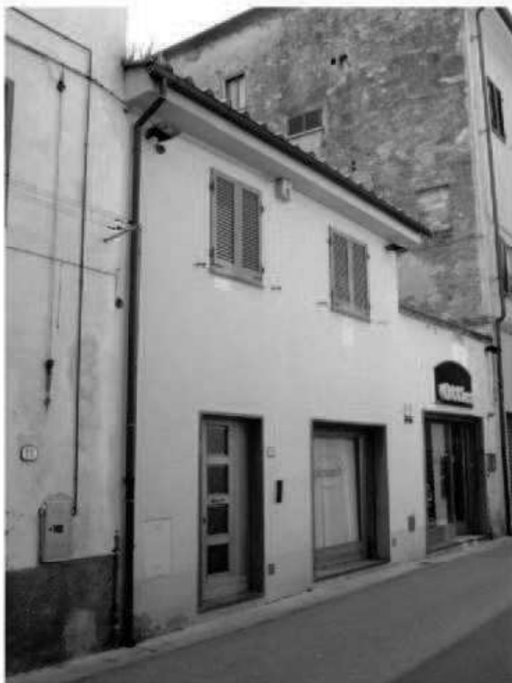
E 10 via Cavour
