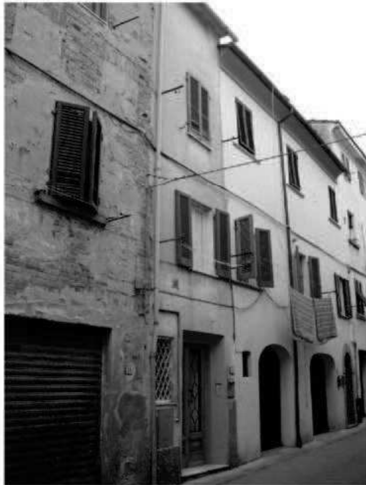
E 6 via Cavour +
