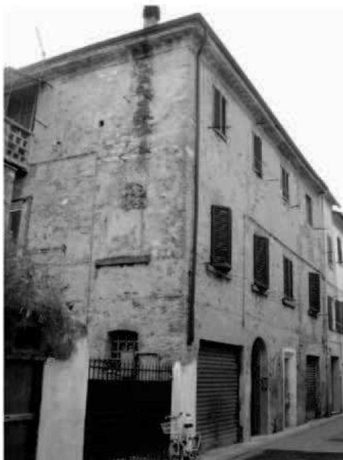
E 4 - via Cavour
