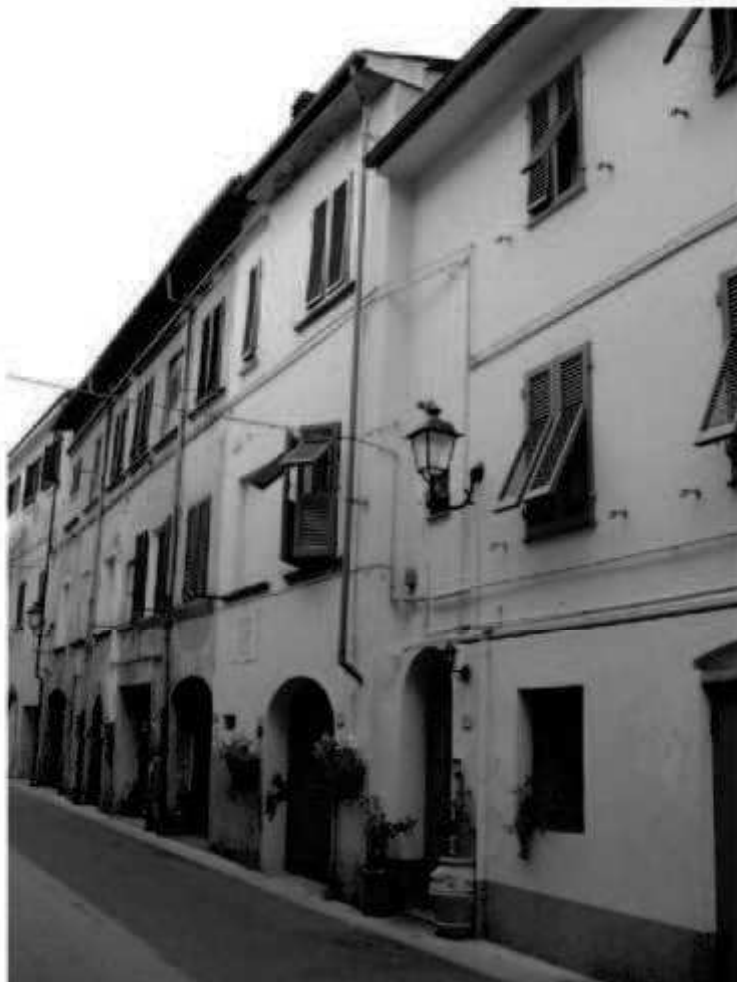
D 6 via Cavour
