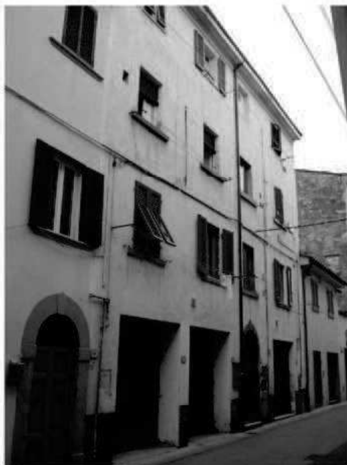
E 9 via Cavour
