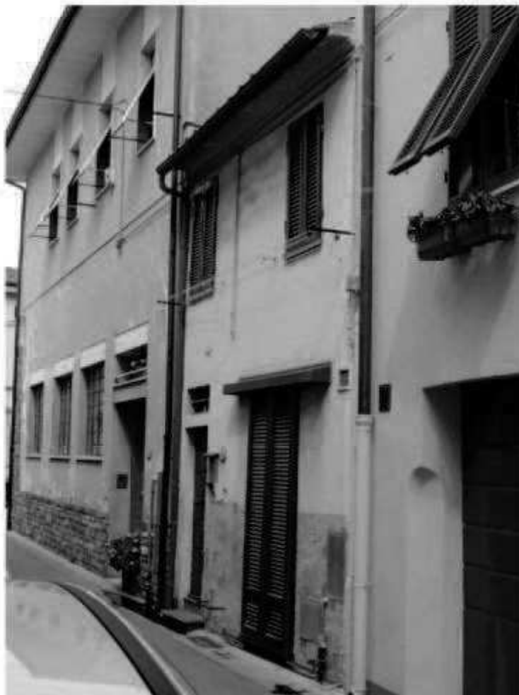
D3 via Cavour
