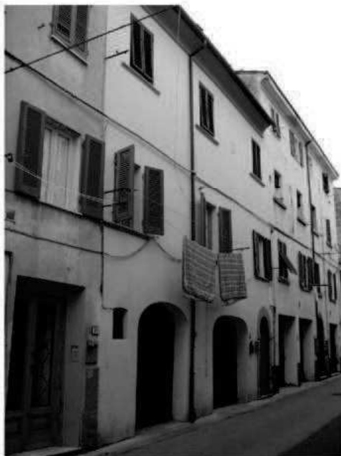
E 8 via Cavour
