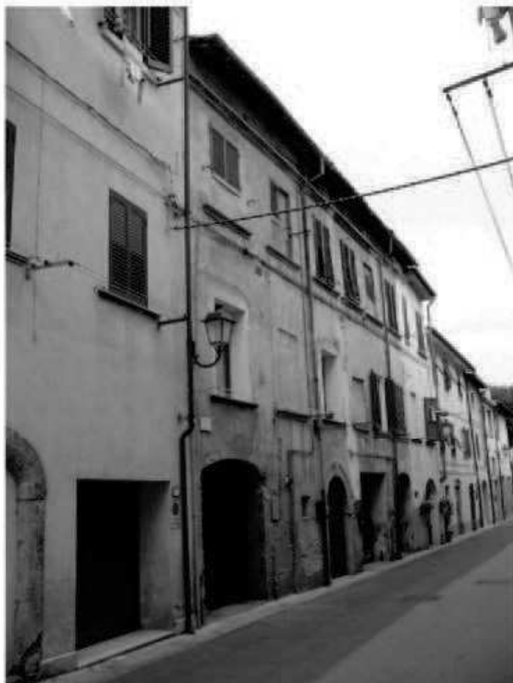
D 2 via Cavour
